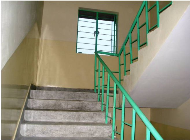
View of the staircase
